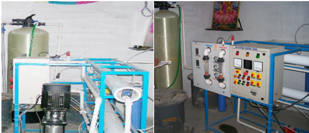
Figure 3 Reverse Osmosis System Control Panel
